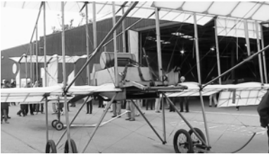
Bristol Boxkite being taken from hangar
